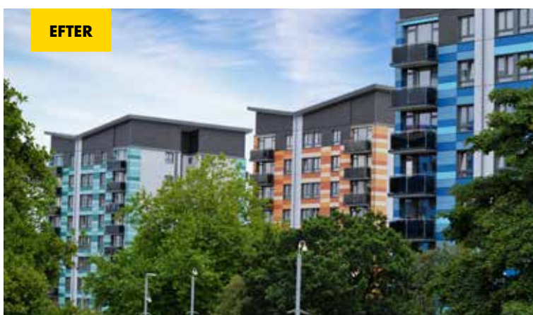
NY FACADEBEKLÆDNING CHARLEMONT FARM ESTATE, UK
