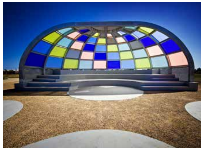
School amphitheatre made of PERSPEX® Frost, Australia ©Photograph: Pavan Consultants / Mitchell Plastics
